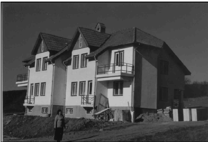
The European Union provided the funding for the Cernatul de Sus orphanage building.
