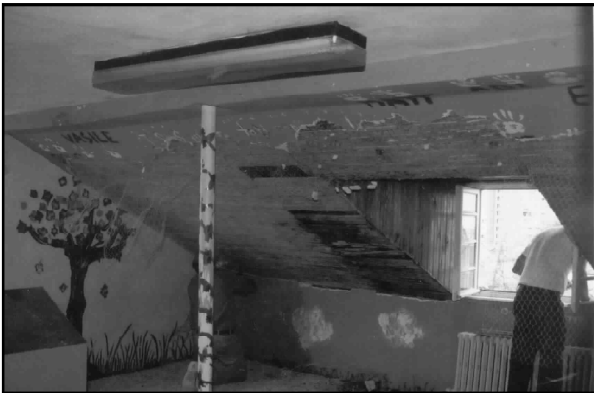
A look at the dayroom under construction
