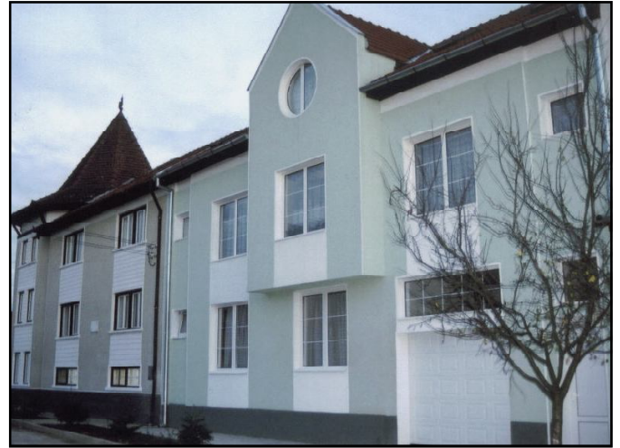
The Alesd Home orphanage built a transition center (green building) next to the orphanage (brown building). Eight fully furnished suites were made for older children who are transitioning to adulthood.
